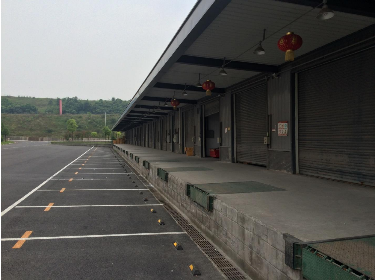
Figure 2: Receiving Dock Bays
