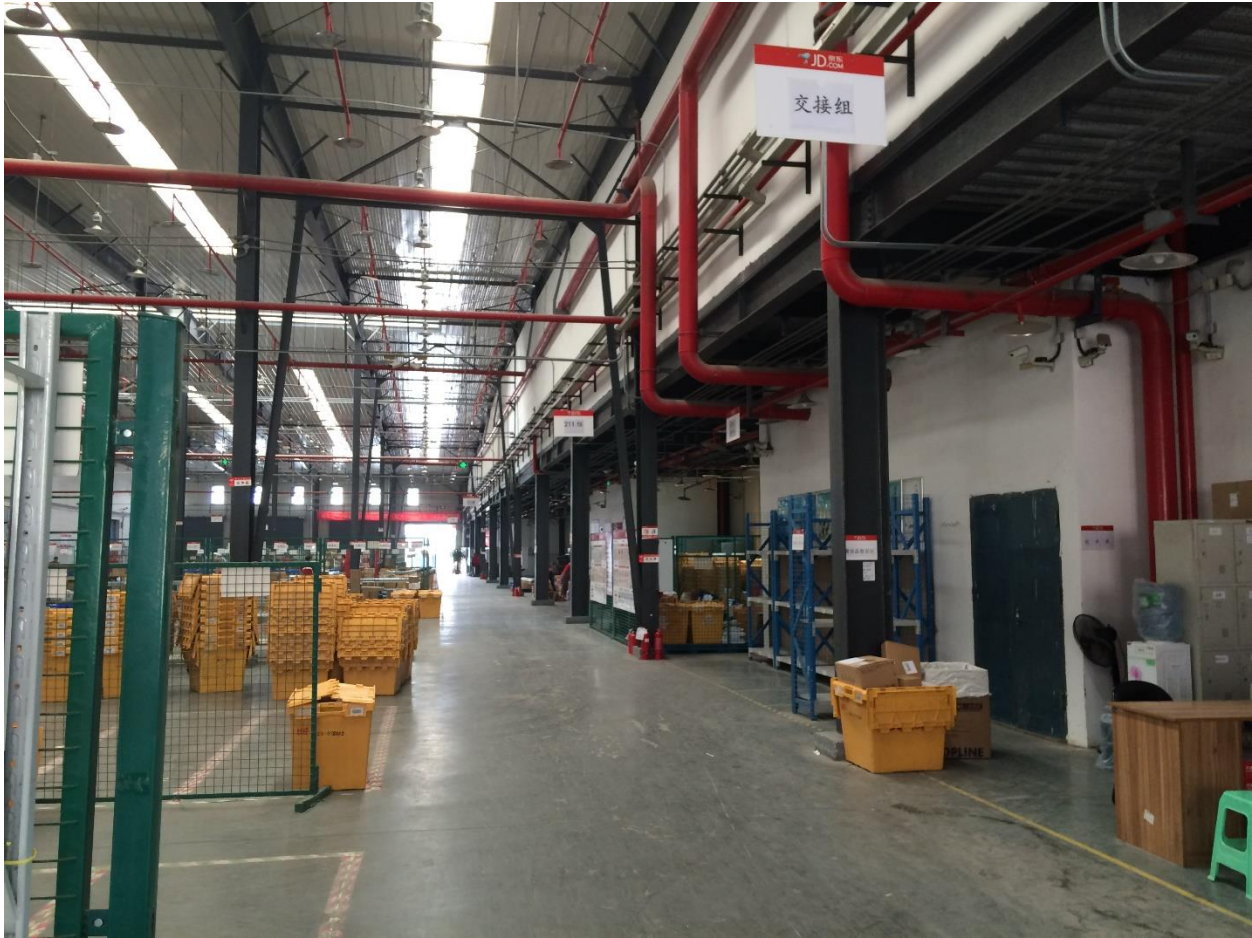
Figure 3: Empty Bins Storage and Preparation Area
