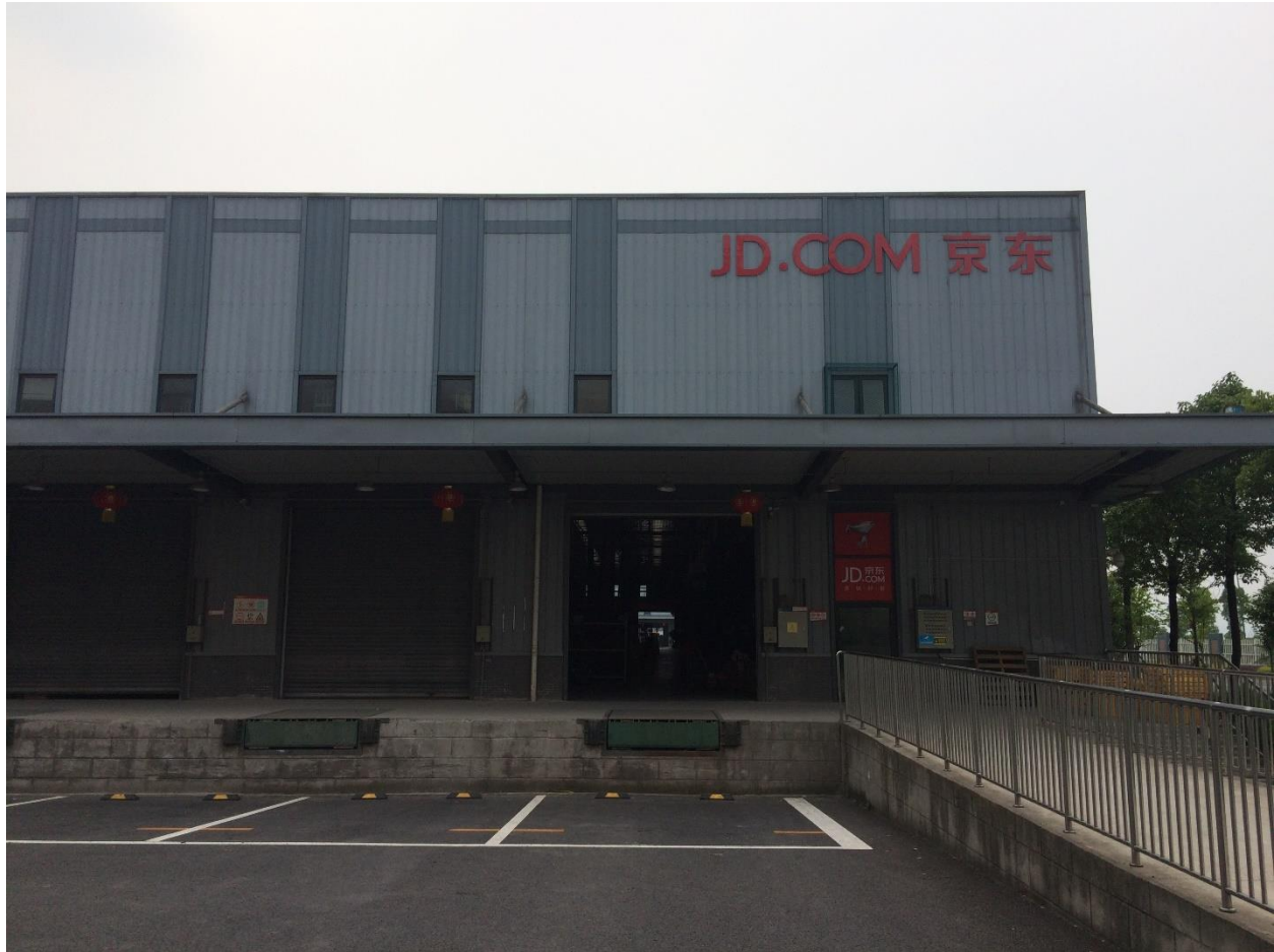
Figure 1: JingDong Distribution Center, Chongqing, China
